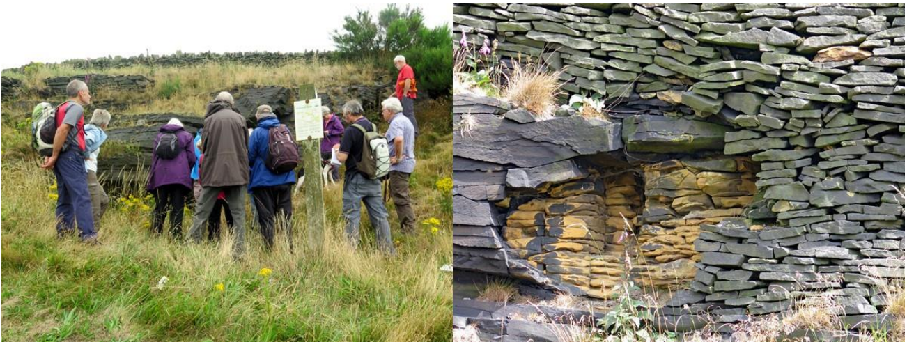
Differential weathering and a fine example of dry stone walling at Don Hill Height quarries
