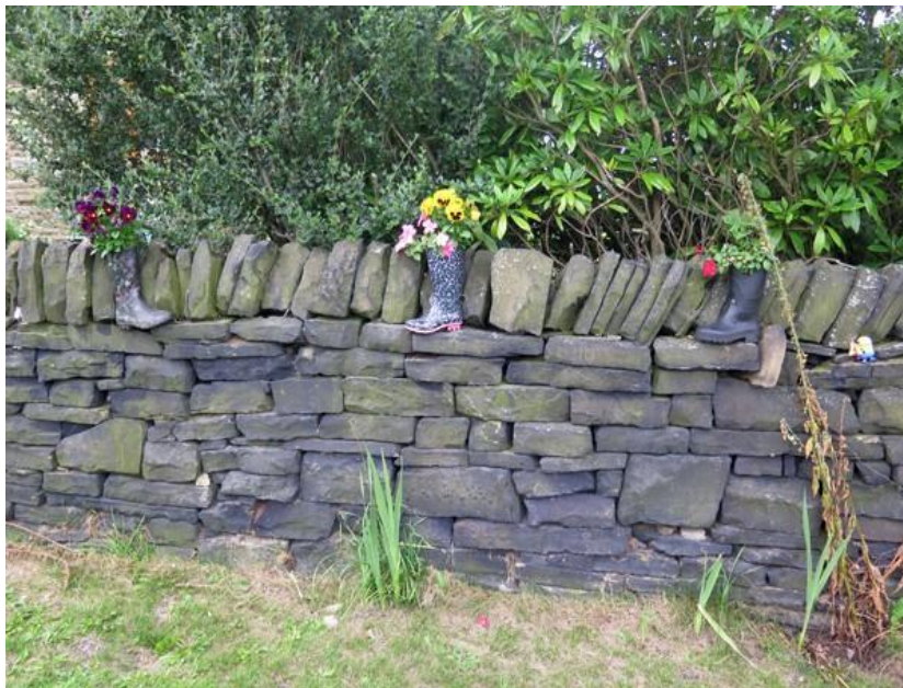
An example of dry stone walling in the Greenmoor Rock
