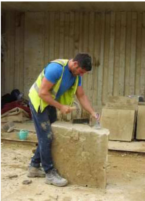
STONE BLOCK BEING SPLIT BY PLUG & FEATHER
